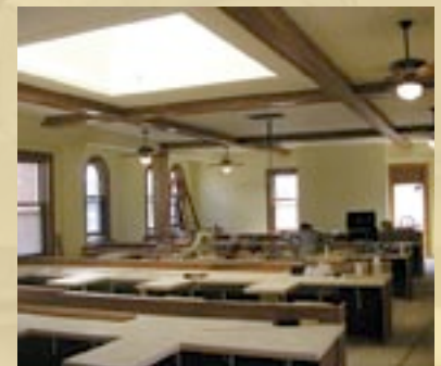
Computer Lab under construction.
