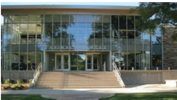
Animal Sciences Building Renovation & Addition
